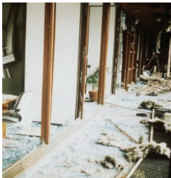
The effect of a blast on toughened glass, bottom picture, compared to laminated glass top picture.
